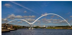
Infinity bridge, Stockton
